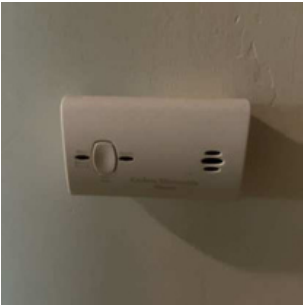
CO / Smoke Detector Battery Check (1/2) 08/21/2023 12:18 PM
