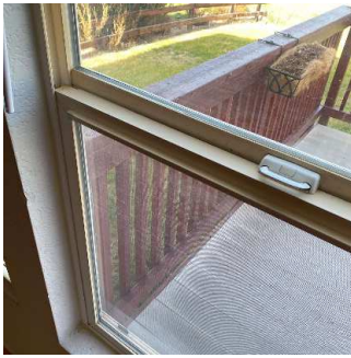
Walls / Windows / Blinds (11/14) 05/11/2020 4:44 PM
