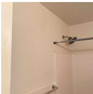
Walls / Windows / Blinds (4/6) 05/11/2020 5:36 PM
