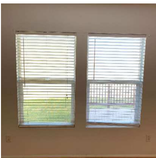
Walls / Windows / Blinds (6/14) 05/11/2020 4:43 PM
