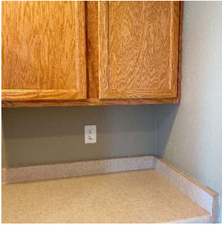
Walls / Windows / Blinds (10/16) 05/11/2020 4:51 PM
