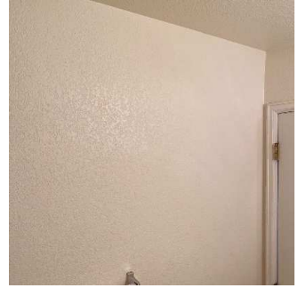
Walls / Windows / Blinds (5/6) 05/11/2020 5:32 PM
