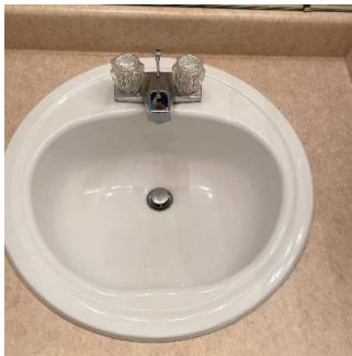
Sink & Underneath Sink (1/3) 05/11/2020 5:37 PM
