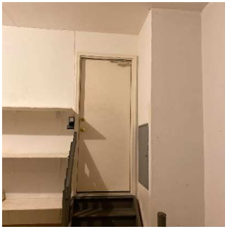
Walls / Windows / Blinds (3/5) 05/11/2020 5:45 PM
