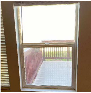
Walls / Windows / Blinds (10/14) 05/11/2020 4:44 PM
