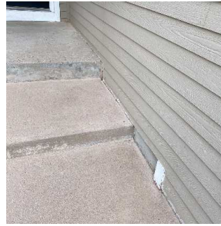
Building Exterior (11/11) 05/11/2020 5:51 PM
