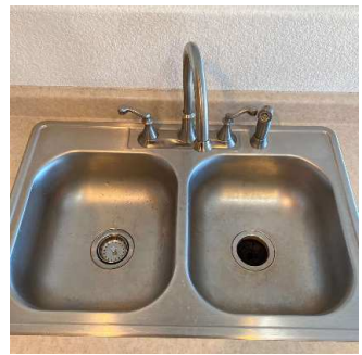
Sink & Underneath Sink (1/4) 05/11/2020 5:02 PM
