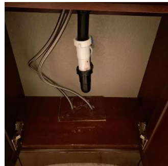
Sink & Underneath Sink (2/2) 05/11/2020 5:10 PM
