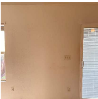
Walls / Windows / Blinds (2/16) 05/11/2020 4:50 PM
