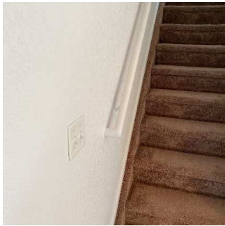
Walls / Windows / Blinds (6/6) 05/11/2020 5:12 PM
