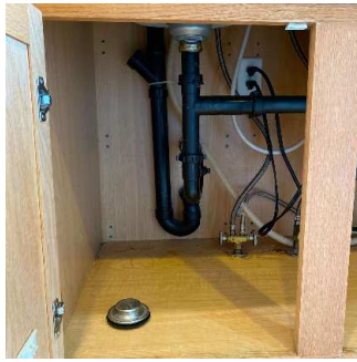
Sink & Underneath Sink (3/4) 05/11/2020 5:02 PM
