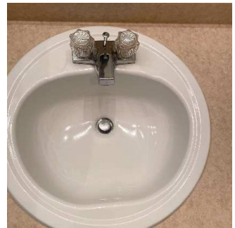
Sink & Underneath Sink (1/3) 05/11/2020 5:33 PM
