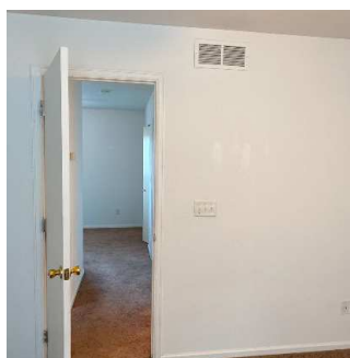
Walls / Windows / Blinds (4/8) 05/11/2020 5:24 PM
