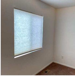
Walls / Windows / Blinds (7/8) 05/11/2020 5:24 PM
