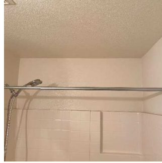
Walls / Windows / Blinds (4/6) 05/11/2020 5:32 PM
