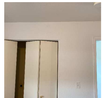
Walls / Windows / Blinds (7/15) 05/11/2020 5:19 PM
