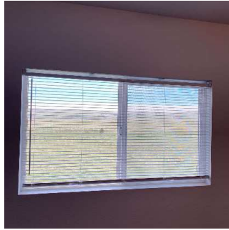
Walls / Windows / Blinds (15/15) 05/11/2020 5:20 PM
