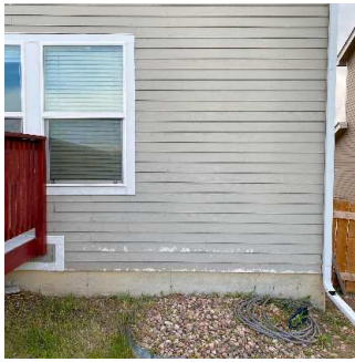
Building Exterior (2/11) 05/11/2020 5:41 PM
