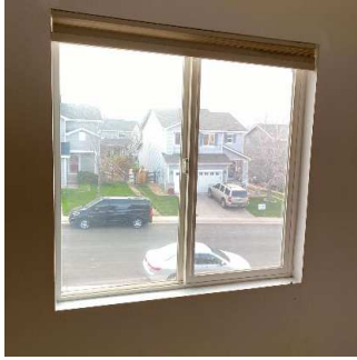
Walls / Windows / Blinds (8/8) 05/11/2020 5:24 PM
