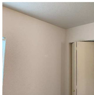
Walls / Windows / Blinds (6/15) 05/11/2020 5:19 PM
