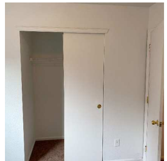
Walls / Windows / Blinds (5/7) 05/11/2020 5:28 PM
