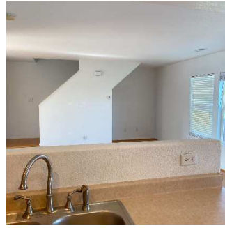
Walls / Windows / Blinds (13/16) 05/11/2020 4:52 PM
