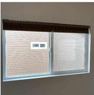
Walls / Windows / Blinds (6/7) 05/11/2020 5:28 PM
