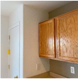
Walls / Windows / Blinds (6/16) 05/11/2020 4:51 PM
