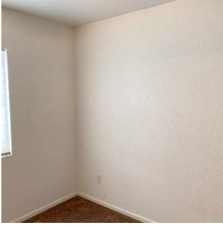
Walls / Windows / Blinds (6/8) 05/11/2020 5:24 PM
