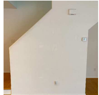
Walls / Windows / Blinds (1/14) 05/11/2020 4:41 PM
