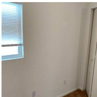
Walls / Windows / Blinds (5/15) 05/11/2020 5:19 PM
