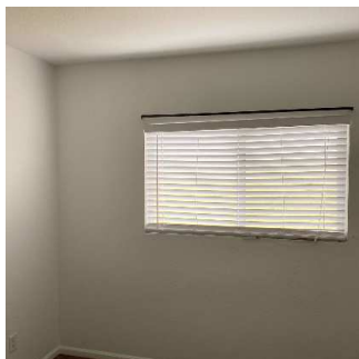
Walls / Windows / Blinds (3/10) 05/11/2020 5:14 PM
