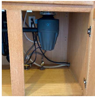
Sink & Underneath Sink (4/4) 05/11/2020 5:02 PM
