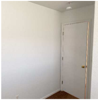
Walls / Windows / Blinds (8/10) 05/11/2020 5:14 PM
