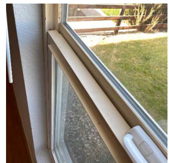
Walls / Windows / Blinds (9/14) 05/11/2020 4:44 PM
