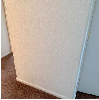
Walls / Windows / Blinds (12/15) 05/11/2020 5:19 PM
