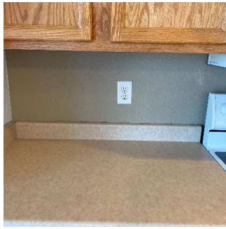
Walls / Windows / Blinds (7/16) 05/11/2020 4:51 PM
