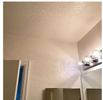
Walls / Windows / Blinds (1/6) 05/11/2020 5:32 PM
