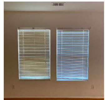
Walls / Windows / Blinds (5/14) 05/11/2020 4:42 PM
