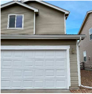
Building Exterior (8/11) 05/11/2020 5:51 PM
