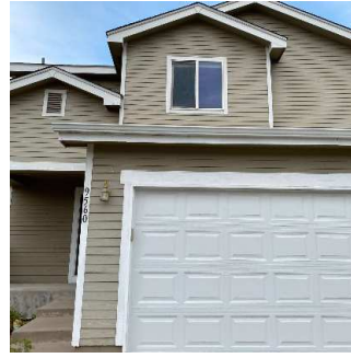
Building Exterior (7/11) 05/11/2020 5:51 PM
