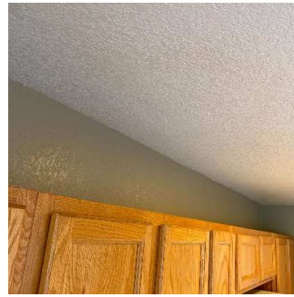
Walls / Windows / Blinds (9/16) 05/11/2020 4:51 PM
