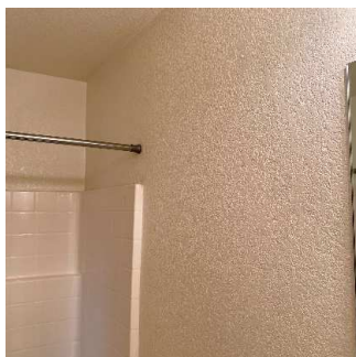
Walls / Windows / Blinds (5/6) 05/11/2020 5:36 PM
