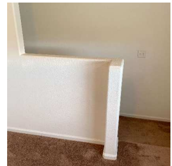
Walls / Windows / Blinds (3/15) 05/11/2020 5:19 PM
