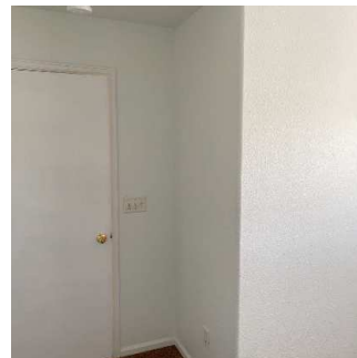
Walls / Windows / Blinds (1/10) 05/11/2020 5:14 PM
