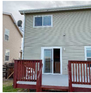
Building Exterior (3/11) 05/11/2020 5:41 PM
