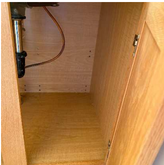
Sink & Underneath Sink (3/3) 05/11/2020 5:37 PM
