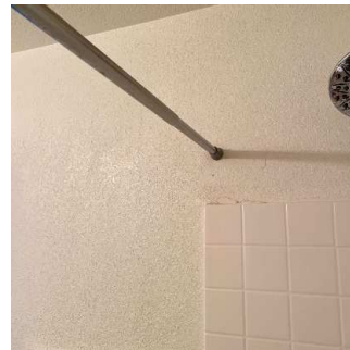
Walls / Windows / Blinds (3/6) 05/11/2020 5:36 PM
