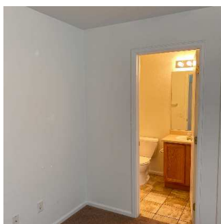
Walls / Windows / Blinds (3/8) 05/11/2020 5:24 PM
