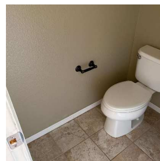
Walls / Windows / Blinds (5/9) 05/11/2020 5:08 PM
