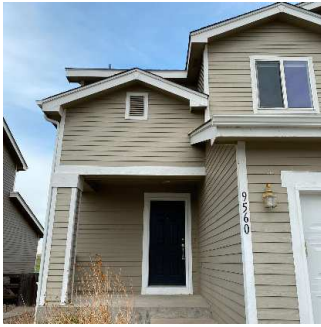
Building Exterior (9/11) 05/11/2020 5:51 PM
