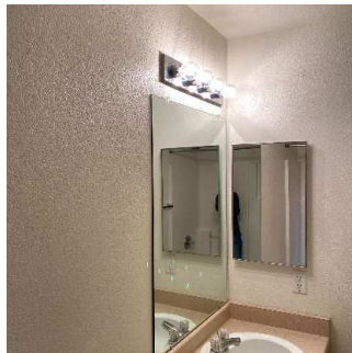
Walls / Windows / Blinds (2/6) 05/11/2020 5:36 PM
