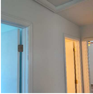
Walls / Windows / Blinds (9/15) 05/11/2020 5:19 PM
