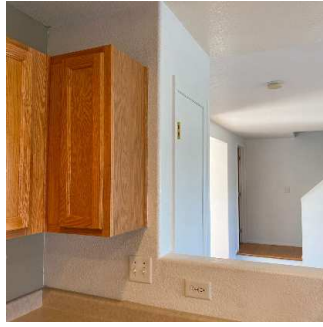
Walls / Windows / Blinds (12/16) 05/11/2020 4:52 PM
