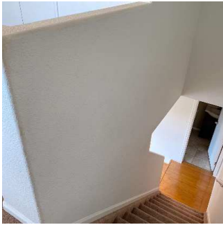
Walls / Windows / Blinds (1/6) 05/11/2020 5:11 PM
