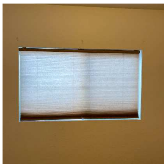
Walls / Windows / Blinds (7/7) 05/11/2020 5:28 PM
