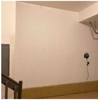
Walls / Windows / Blinds (4/5) 05/11/2020 5:45 PM
