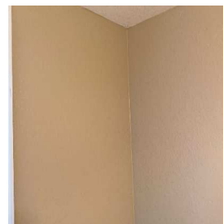
Walls / Windows / Blinds (1/9) 05/11/2020 5:08 PM
