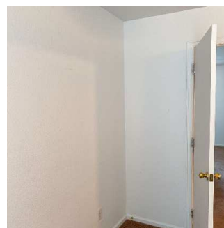
Walls / Windows / Blinds (5/8) 05/11/2020 5:24 PM
