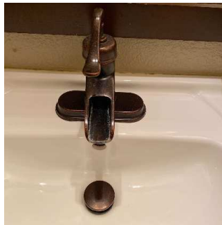
Sink & Underneath Sink (1/2) 05/11/2020 5:10 PM
