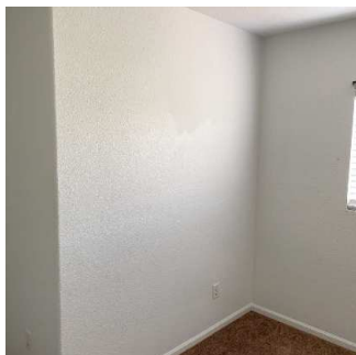
Walls / Windows / Blinds (2/10) 05/11/2020 5:14 PM
