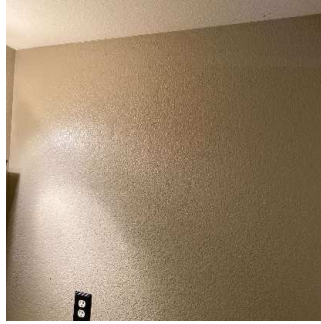
Walls / Windows / Blinds (8/9) 05/11/2020 5:09 PM
