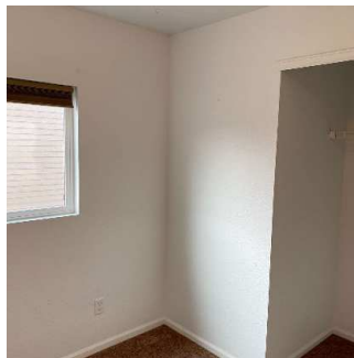
Walls / Windows / Blinds (4/7) 05/11/2020 5:28 PM
