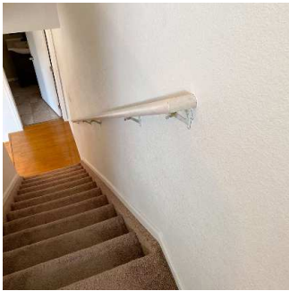
Walls / Windows / Blinds (4/6) 05/11/2020 5:12 PM
