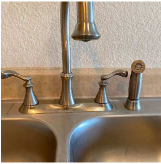
Sink & Underneath Sink (2/4) 05/11/2020 5:02 PM
