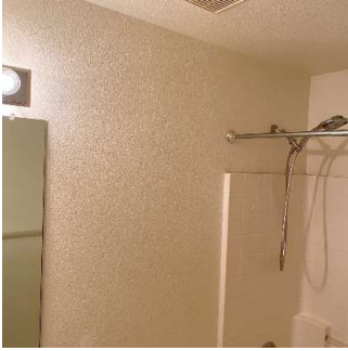
Walls / Windows / Blinds (2/6) 05/11/2020 5:32 PM
