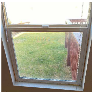
Walls / Windows / Blinds (7/14) 05/11/2020 4:43 PM
