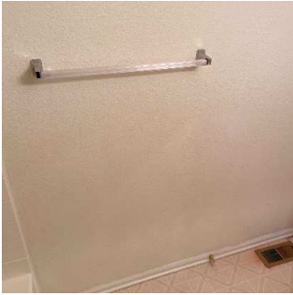
Walls / Windows / Blinds (6/6) 05/11/2020 5:32 PM
