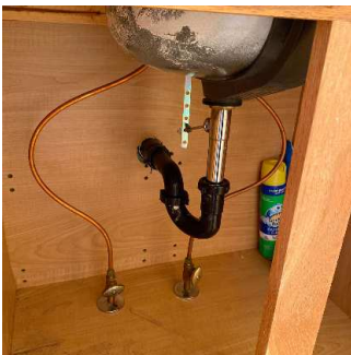
Sink & Underneath Sink (2/3) 05/11/2020 5:34 PM
