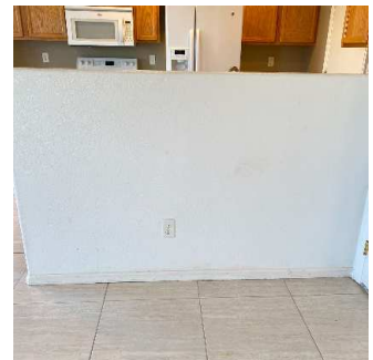
Walls / Windows / Blinds (1/16) 05/11/2020 4:50 PM
