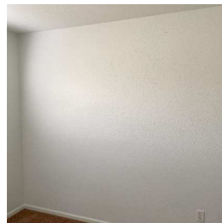
Walls / Windows / Blinds (5/10) 05/11/2020 5:14 PM
