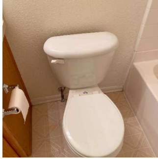
Walls / Windows / Blinds (3/6) 05/11/2020 5:32 PM
