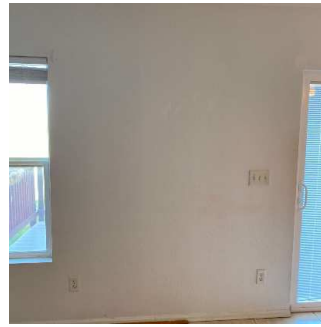
Walls / Windows / Blinds (13/14) 05/11/2020 4:44 PM
