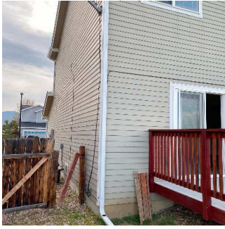
Building Exterior (5/11) 05/11/2020 5:42 PM
