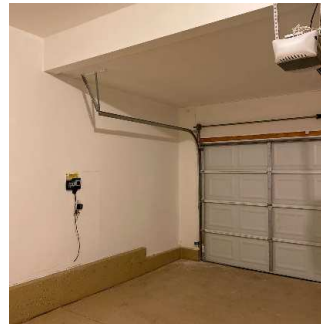
Walls / Windows / Blinds (5/5) 05/11/2020 5:45 PM
