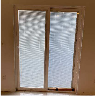
Walls / Windows / Blinds (14/16) 05/11/2020 4:52 PM
