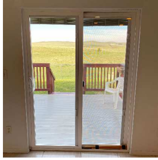
Walls / Windows / Blinds (16/16) 05/11/2020 4:53 PM
