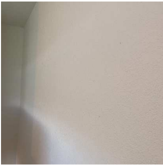
Walls / Windows / Blinds (3/6) 05/11/2020 5:12 PM
