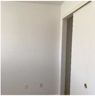
Walls / Windows / Blinds (6/10) 05/11/2020 5:14 PM
