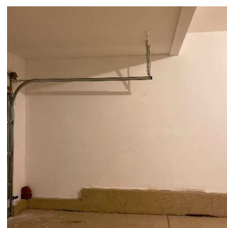
Walls / Windows / Blinds (1/5) 05/11/2020 5:45 PM
