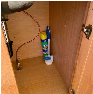
Sink & Underneath Sink (3/3) 05/11/2020 5:34 PM
