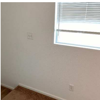
Walls / Windows / Blinds (4/15) 05/11/2020 5:19 PM
